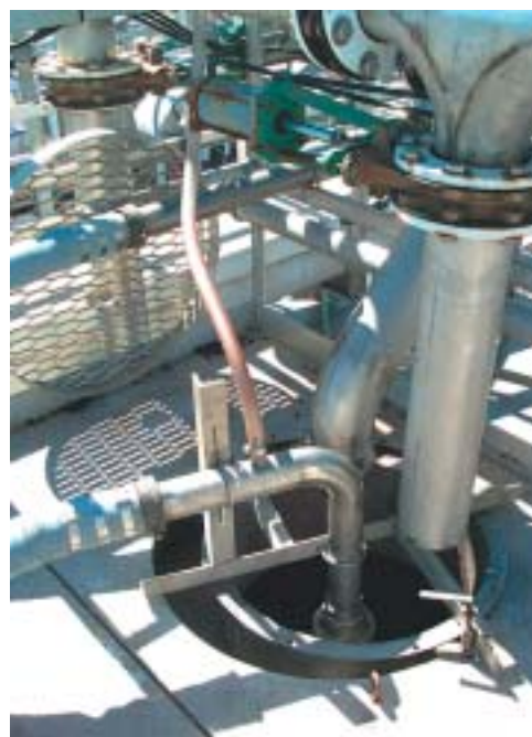
Irrigator with venturi in place. A venturi can also be used to induce more efficient aeration during racking.
